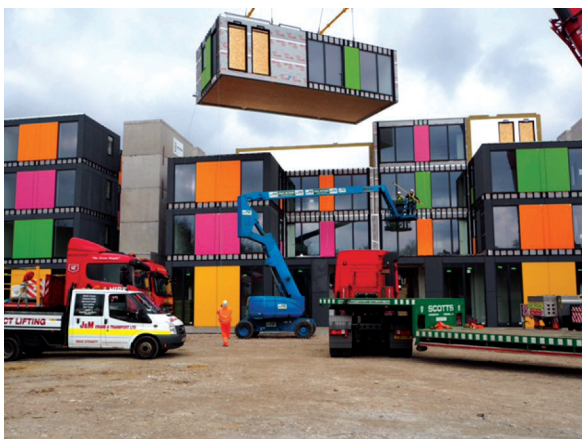
Ladywell development, exterior
